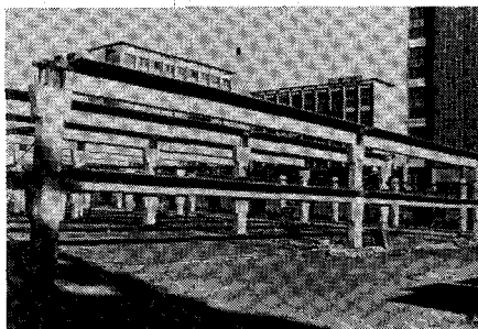
Structure after columns and girders had been erected.
